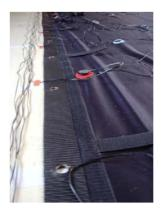
When you're finished doing this, and all the cables are marked and placed next to each other, you can divide the positive and negative wire from the cable. You can do this quite easily by cutting a small incision with the wire cutter and pull the wires further from each other for another 10 cm. The negative pole can be recognized by the dotted line, the positive pole is marked with some text.
