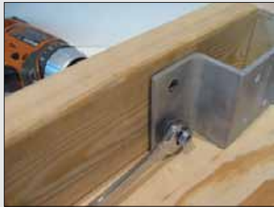
Bolt to unit using 3/8" flat head stove bolts, Nylock nuts, and washers.
