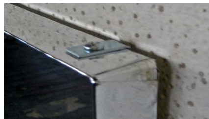
Hidden Bracket (Holes are located 1 \frac{1}{8} " from the corner)
