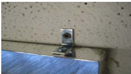
Visible Bracket (Holes are located 1 \frac{9}{16} " from the corner)
