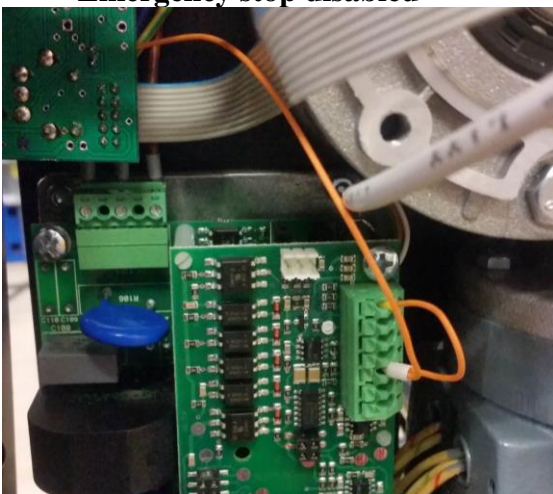
Emergency stop disabled
